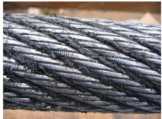
Effect of system gripping on wire under 180Te test load
