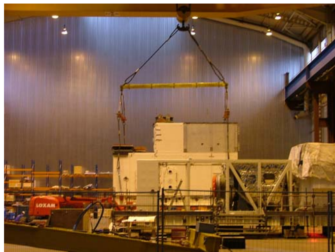
Lift Arrangement Using Modular Lifting Beams
