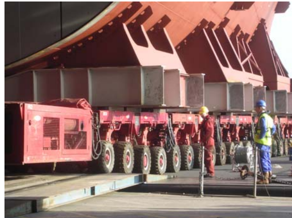
Figure 13: Hydraulic Self-Elevating Trailers during loadout
